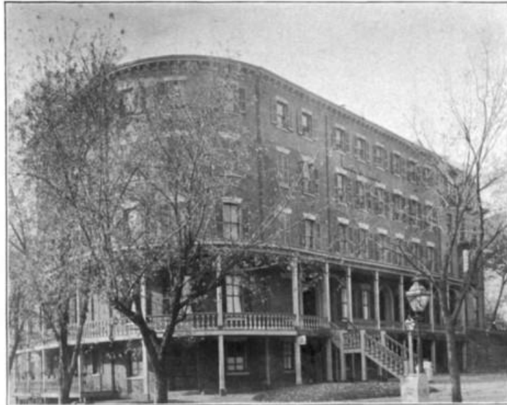
Conrad and McMunn’s boarding house where Marshall and the justices first boarded ca 1801.
