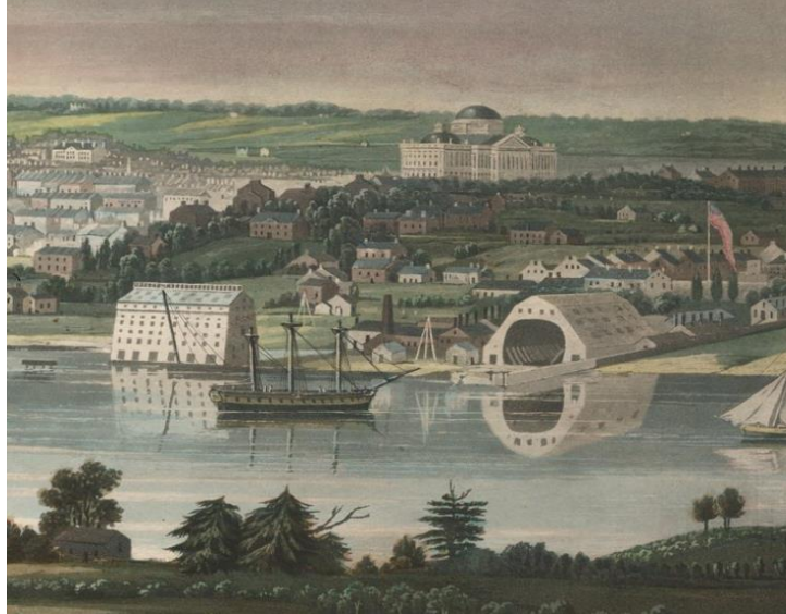
View of Washington from beyond the Navy Yard by George Cooke, 1834. The ropewalk would have been to the left of the dock area.
